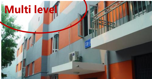
The first all-graded aggregate recycled concrete test building in China
