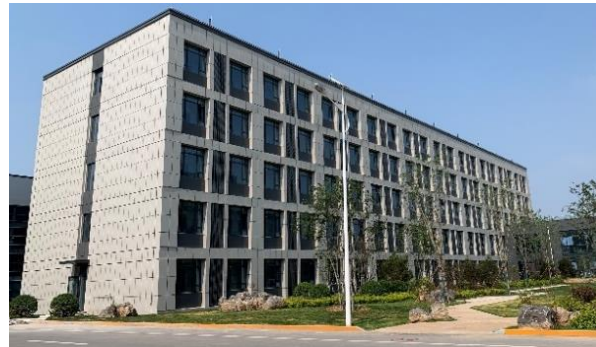
Jinan, 5-floor large-span framework, 2020 (with a 100% replacement rate)
