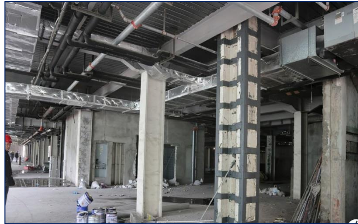
Original demolished materials
