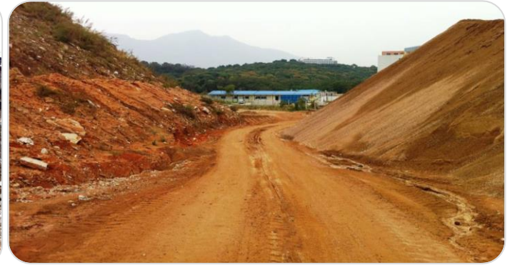
The Left Side Shows Untreated Construction Waste The Right Side Shows Treated Recycled Fine Aggregate
