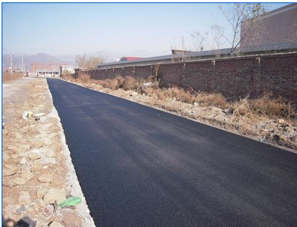
Recycled Aggregate Base Test Road Used for 14 Years Without Any Issues
