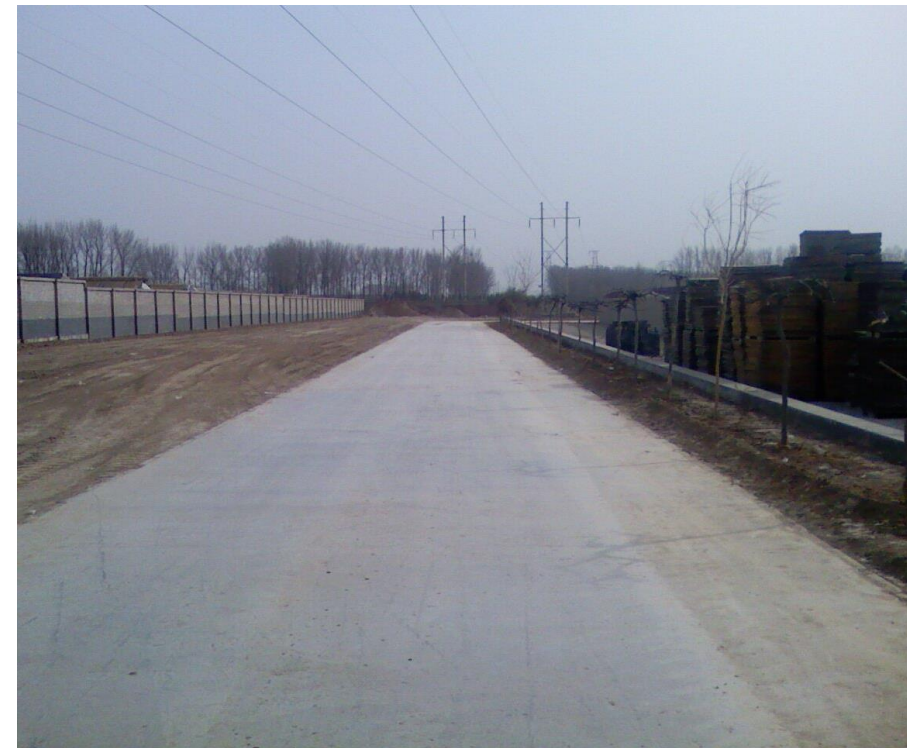
Recycled Concrete Test Road Used for 15 Years
