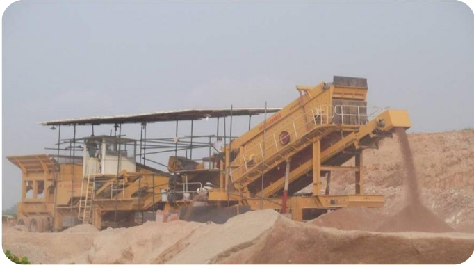
On-site Crushing Treatment
